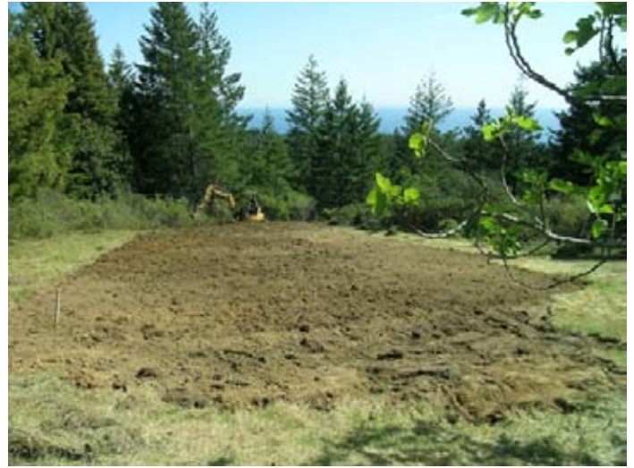
Fig. 6. The site for the wave meander earthwork after preparation
